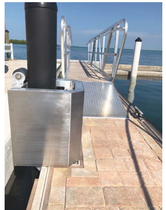
Protective Cowling Constructed with 6061-T6 Aluminum
