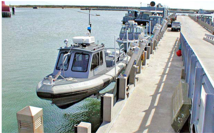
Client: Texas Navy Base Products: (3) Elevator Lifts
