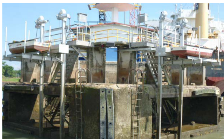
Client: Republic of Panama Brief: Due to the extreme water rise in the lock, the Elevator Lifts travel 30' - double what is typically needed. Because of this, everything about the project is oversized and overbuilt.
